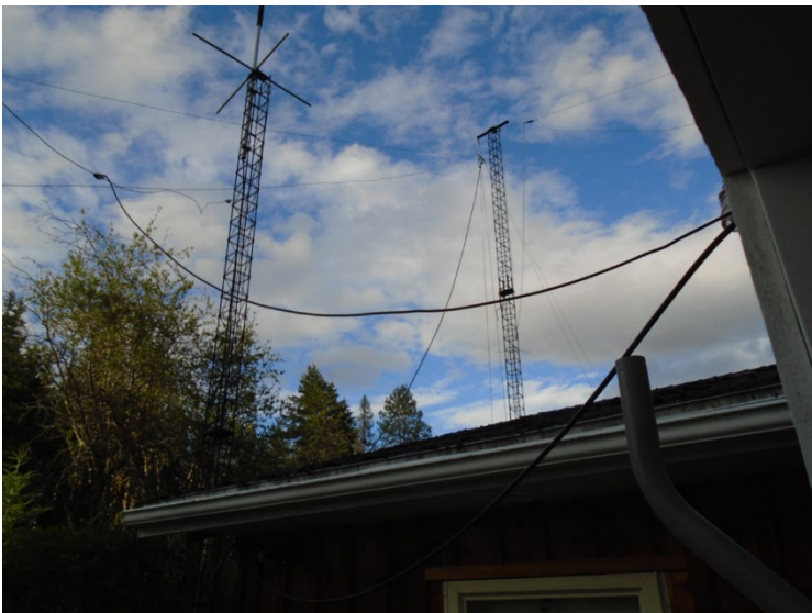
The antenna farm showing the long wire and the dipole I sometimes use.
